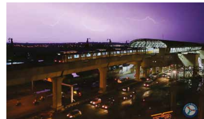
100% LED Lit Stations & Trains
