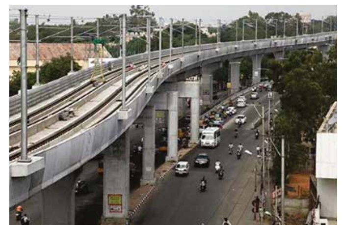
Rain water harvesting of Run-off from stations & viaduct
